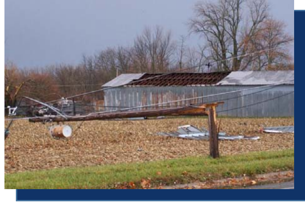
An EF 2 tornado on November 17, 2013 snapped power poles and damaged roofs.
