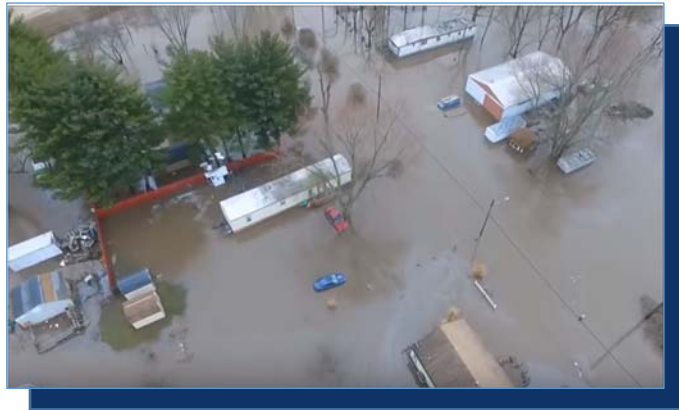
Morin’s Addition on the west side of Danville experienced riverine flooding in February 2018.
